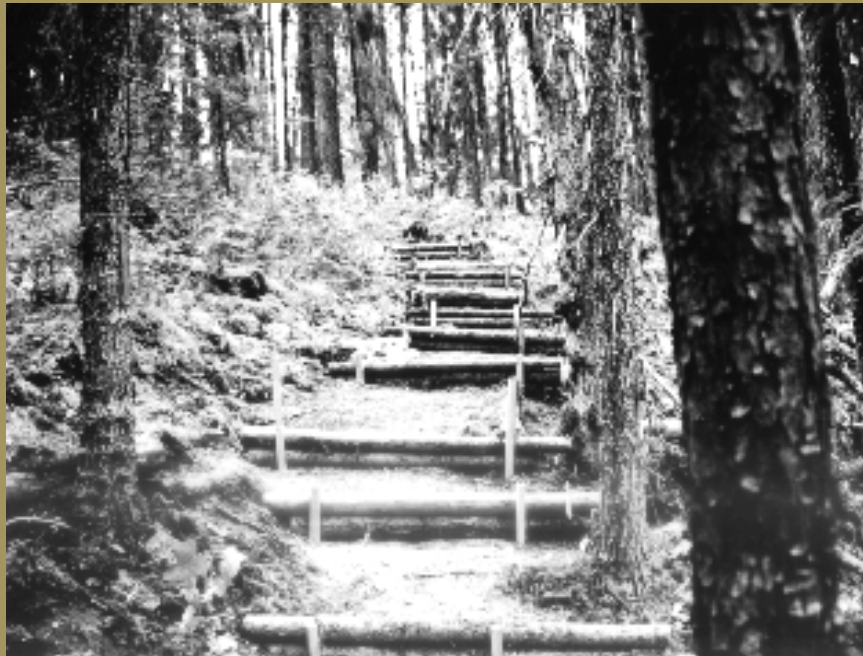
Stairs made from local material help the trail retain a rustic appearance and prevent erosion.
